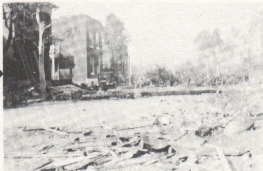
'27 Tornado removes front wall of flat minutes after Ilda's Mom leaves room
